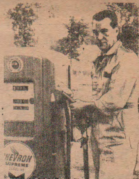
AT THE PUMPS
