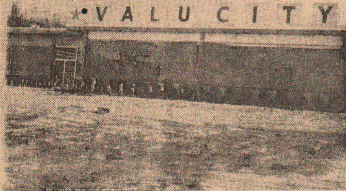
SHEETS OF PLYWOOD, HASTILY NAILED UP, COVER THE BROKEN WINDOWS OF THE VALU CITY STORE AT THE EAGLE RIVER SHOPPING CENTER. ONE OF THE MOST HEAVILY HIT OF THE LOCAL BUILDINGS BY LAST FRIDAY'S EARTHQUAKE.
