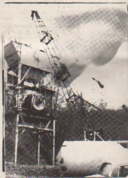
TIL'S TOWER, ON THE WAY UP!
