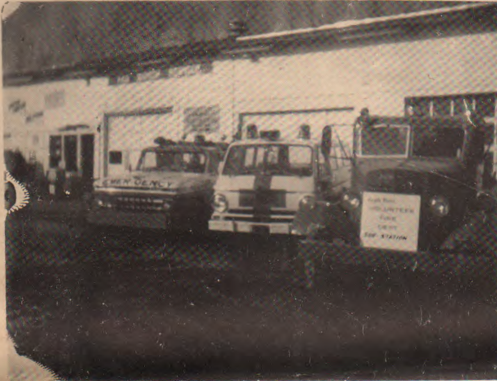
EAGLE RIVER FIRE EQUIPMENT LINES UP IN FRONT OF THE NEW SUB-STATION AT FAR NORTH SERVICE.
