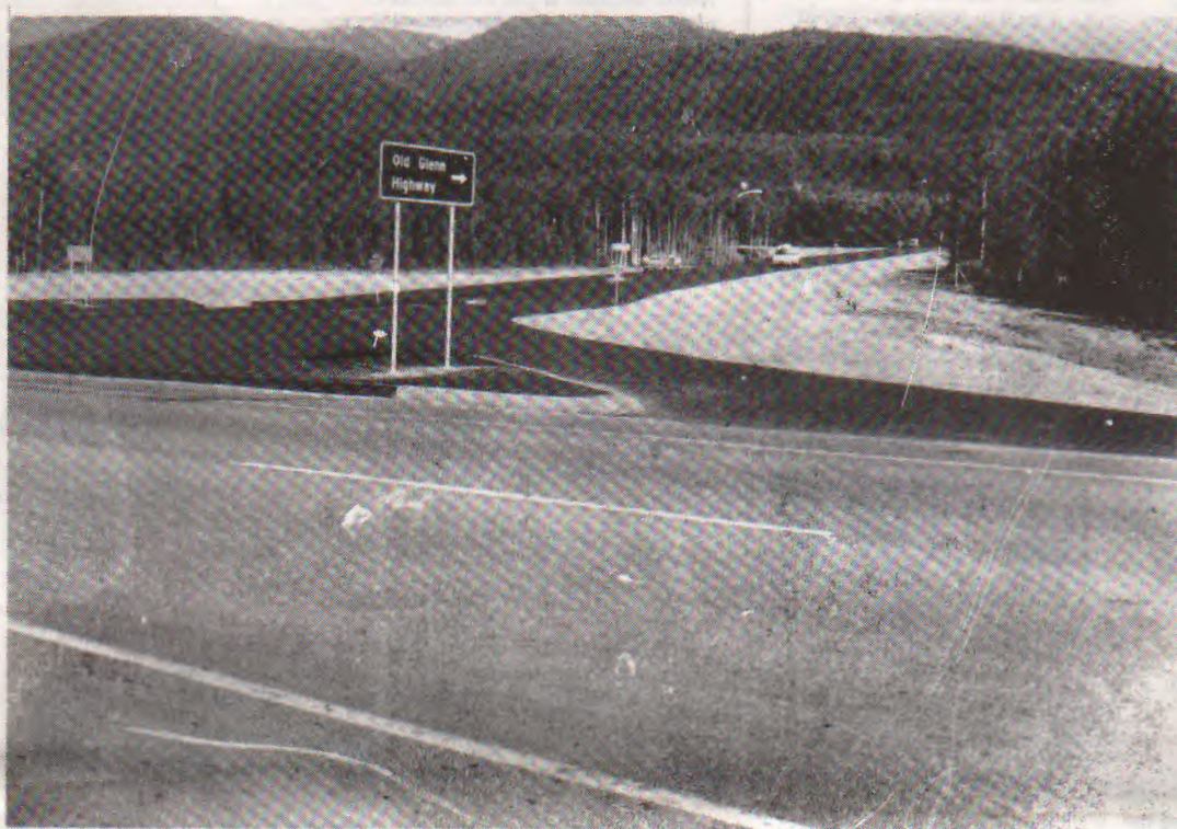
NEW "NORTH EAGLE RIVER ACCESS ROAD" OPENS TO TRAFFIC THIS WEEK.
