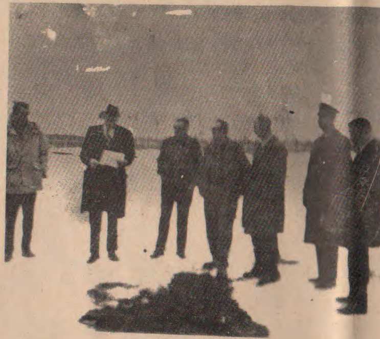
BOROUGH CHAIRMAN, JOHN ASPLUND READS A LETTER FROM GOVERNOR EGAN APOLOGIZING FOR BEING UNABLE TO ATTEND THE DEDICATION OF THE EAGLE RIVER SEWER SYSTEM.
